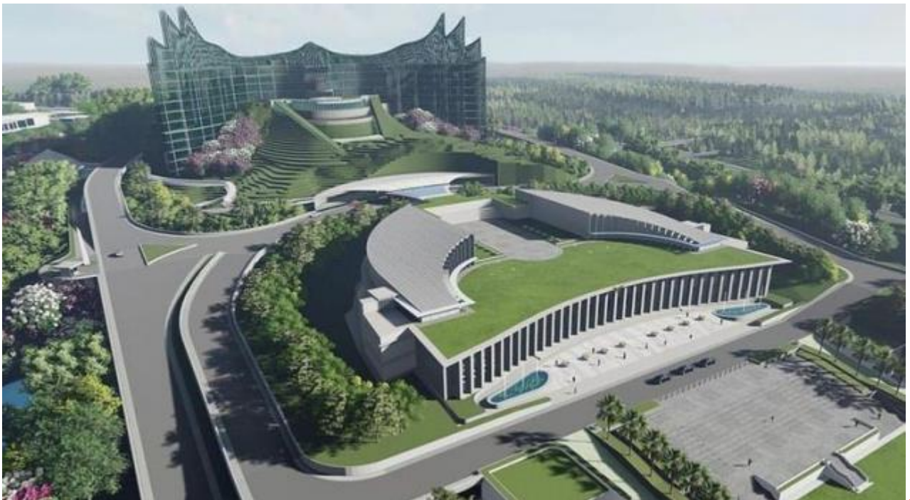
Indonesia New Capital Nusantara Project Keep On Progress
