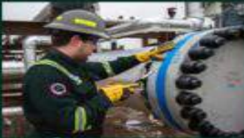
Process pre-commissioning and commissioning
